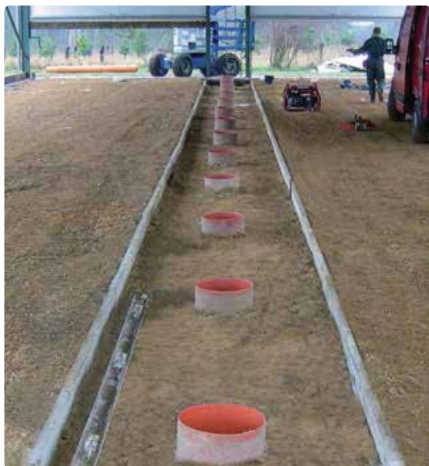
Preparation for pouring of concrete
