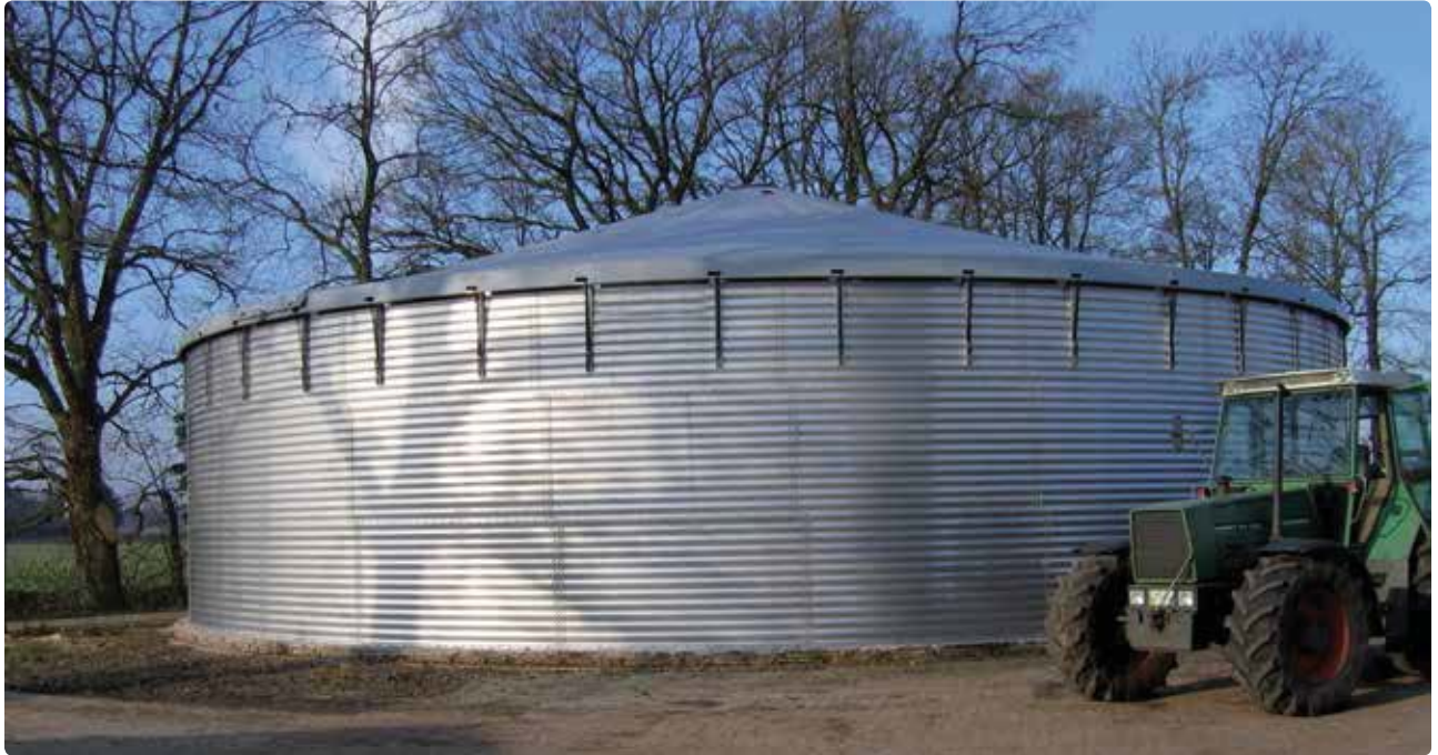
Corrugated high-grade steel container with foil covering
