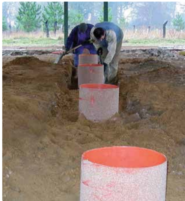
Manual infilling and soil compaction
